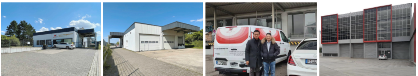
@ Sunstone Power Industrial GmbH
